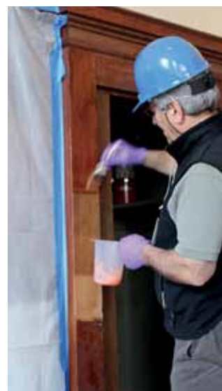
Conservator Sally Malenka examines a gallery wall in the Rodin Museum; conservator Behrooz Salimnejad conducts testing for finishing the library woodwork at the Rodin Museum.
