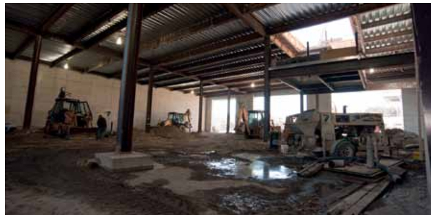
The Museum's new Art Handling Facility during construction
