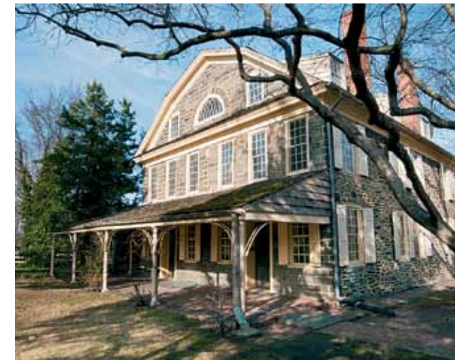
Cedar Grove historic house in Fairmount Park
